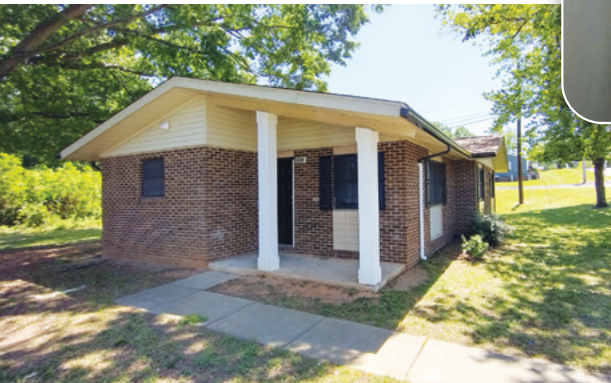
1200 Boyte Exterior Side (new columns)
